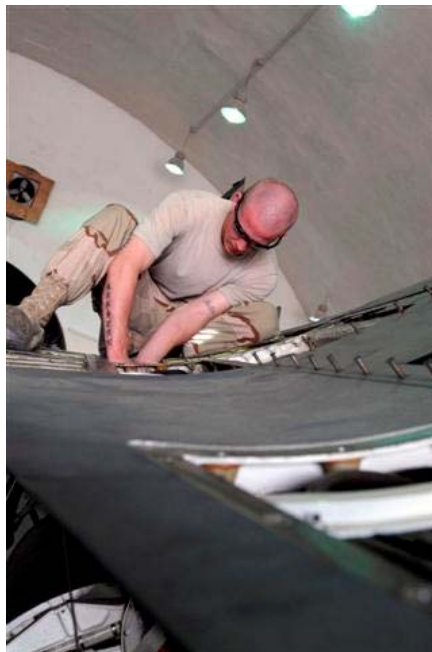
Figure 6. Repair Requiring Elevated Panel Removal (Air Force, Photos, 2008)
